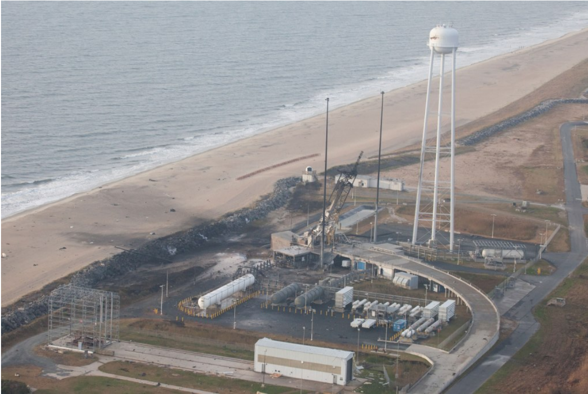
Figure 2. Antares Launch Pad Damage Following the Orb-3 Accident
